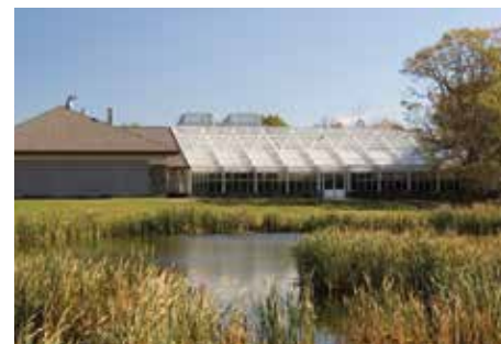
NEB's unique wastewater treatment facility treats the campus' wastewater for groundwater recharge.
