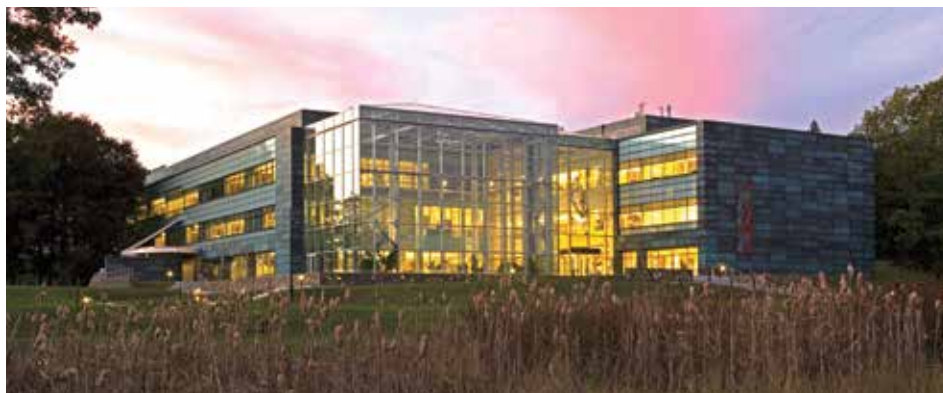
NEB Headquarters in Ipswich, MA, is LEED-certified and designed with sustainability in mind.
